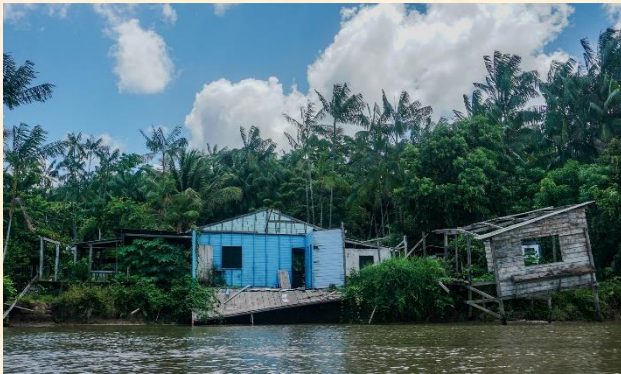
Abandoned houses at the south of the archipelago about to fall due to the erosion of the Amazon River. Residents first take out parts of the houses so they can be reused to build a new house. Image by Rudja Santos.
