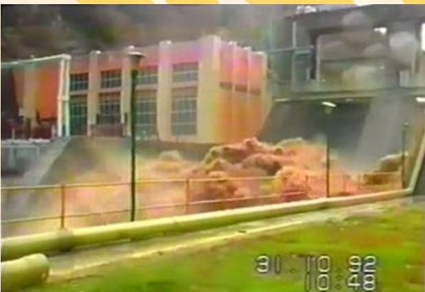
Levane Dam during the flood event of October 1992
