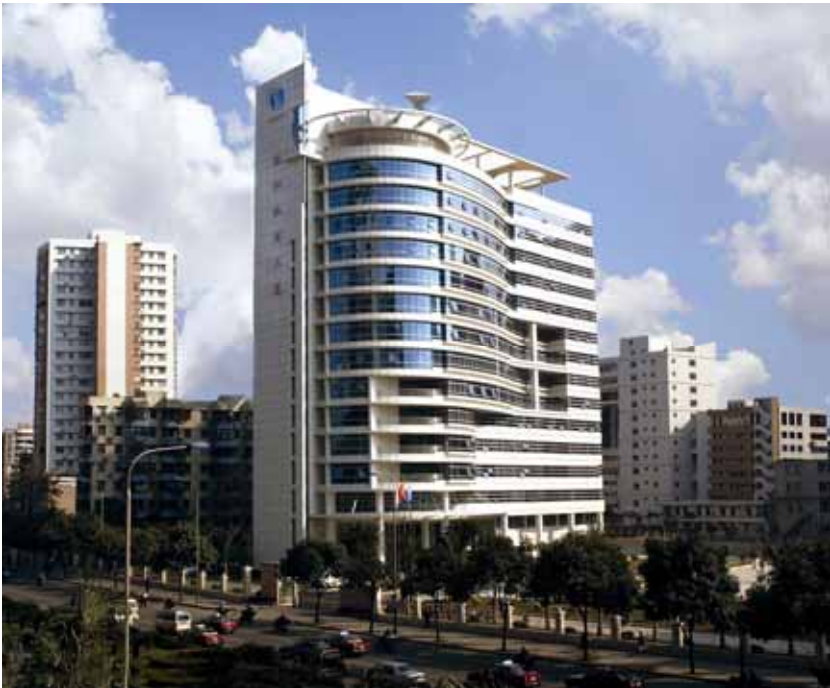
Pearl River Water Resources Commission Headquarter
